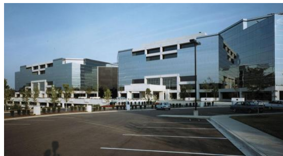
Figure 6: Towers of Kenwood
